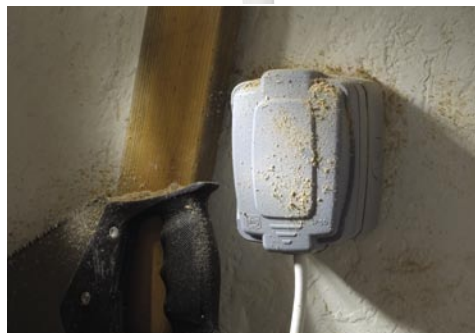
Dust proof connection to safeguard work areas.
