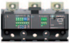
Loose trip units
