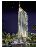
Skyview tower UAE
